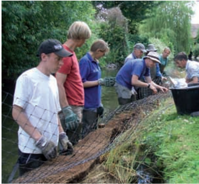
Volunteers help to create natural river banks (Living River).
